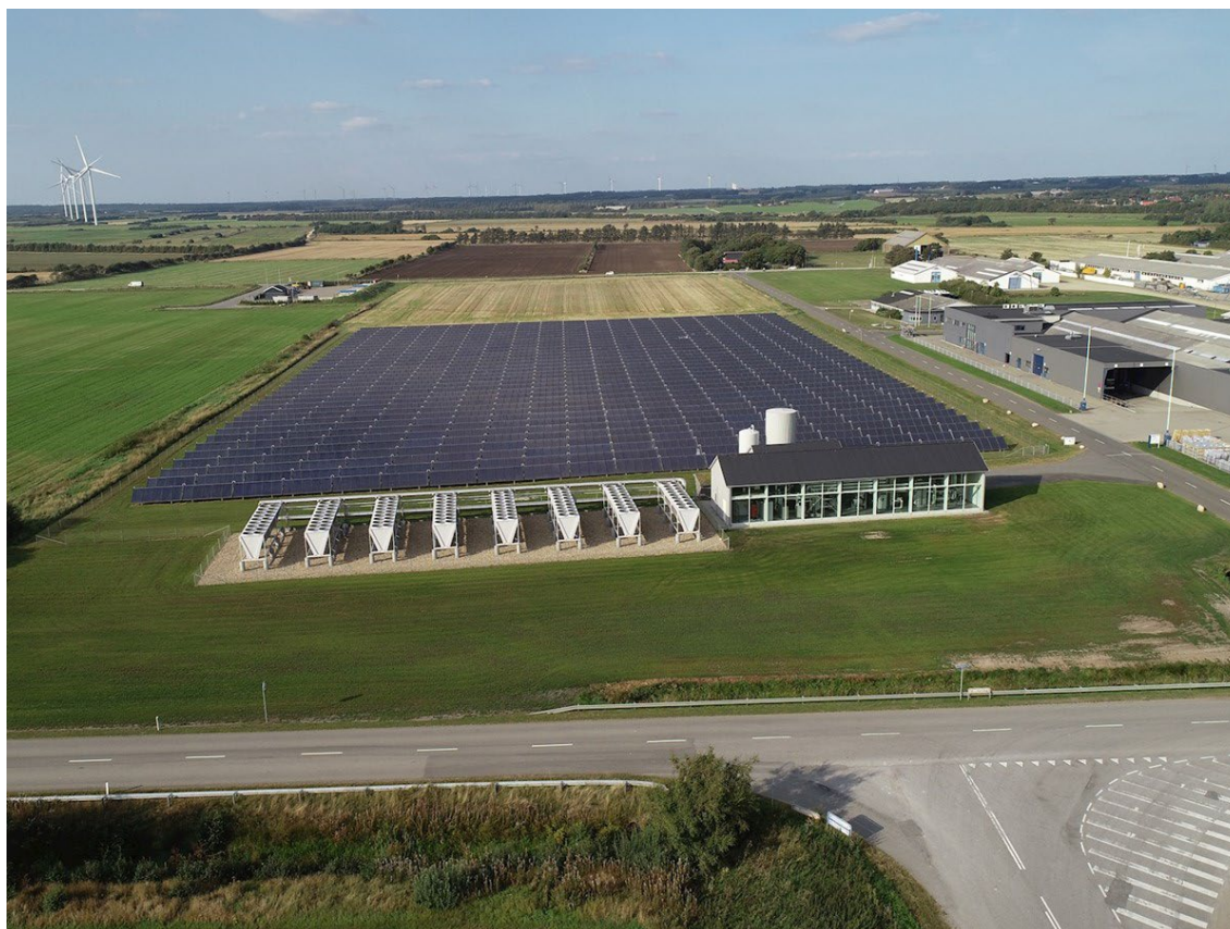
Slika 14: Lem district heating plant
